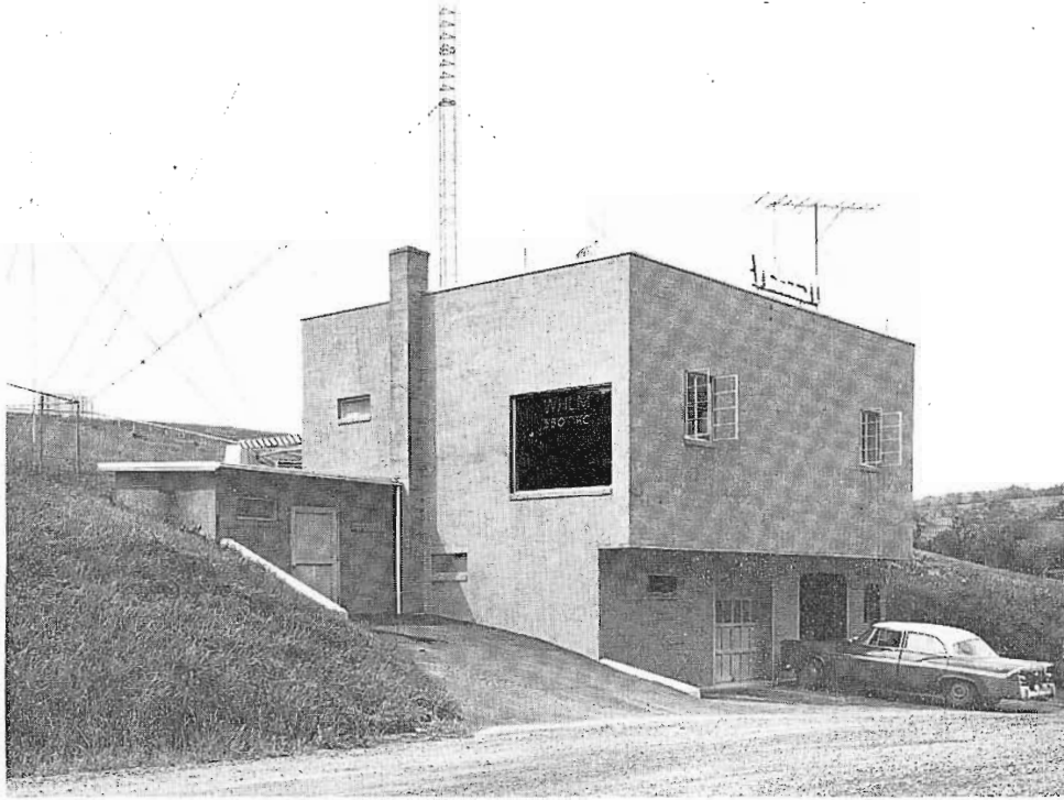
FIG. 5. The WHLM transmitter building lies in the valley between the second and third tower. It is constructed of concrete block and has more-than-adequate room for its AM and FM transmitting equipment.
